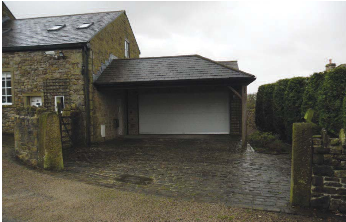
Garage (23'0" x 20'0") with concrete floor, Garog electric operated fold up aluminium door, single door entrance, rear sliding door to the workshop, three double fluorescent ceiling lights and three double power points.
